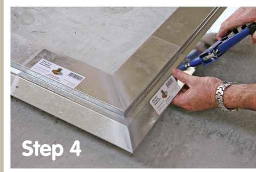
Step 4 Internal and external corners are formed as EZI as that. Once position is confirmed corners can be pop riveted to straight sections if required.
