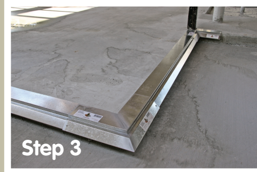
Step 3 The next corner cap is then laid over the following section to form the preceding corner.
