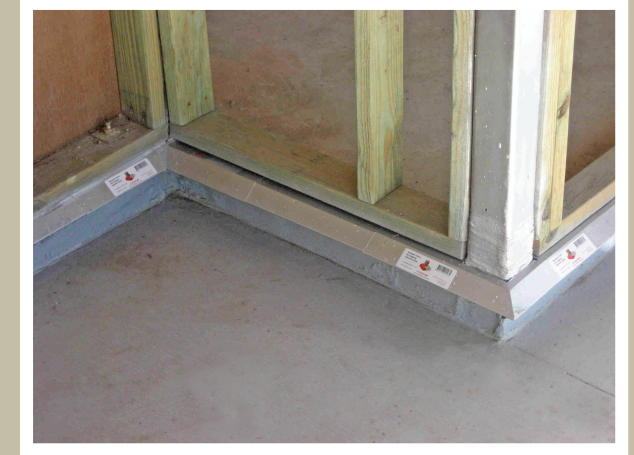
Suitable for use on either slab on ground or with combination of slabs & steel columns as corners are welded.
